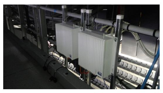
Two remote units are deployed on the catwalk to help ensure powerful cellular coverage is available throughout the arena.
